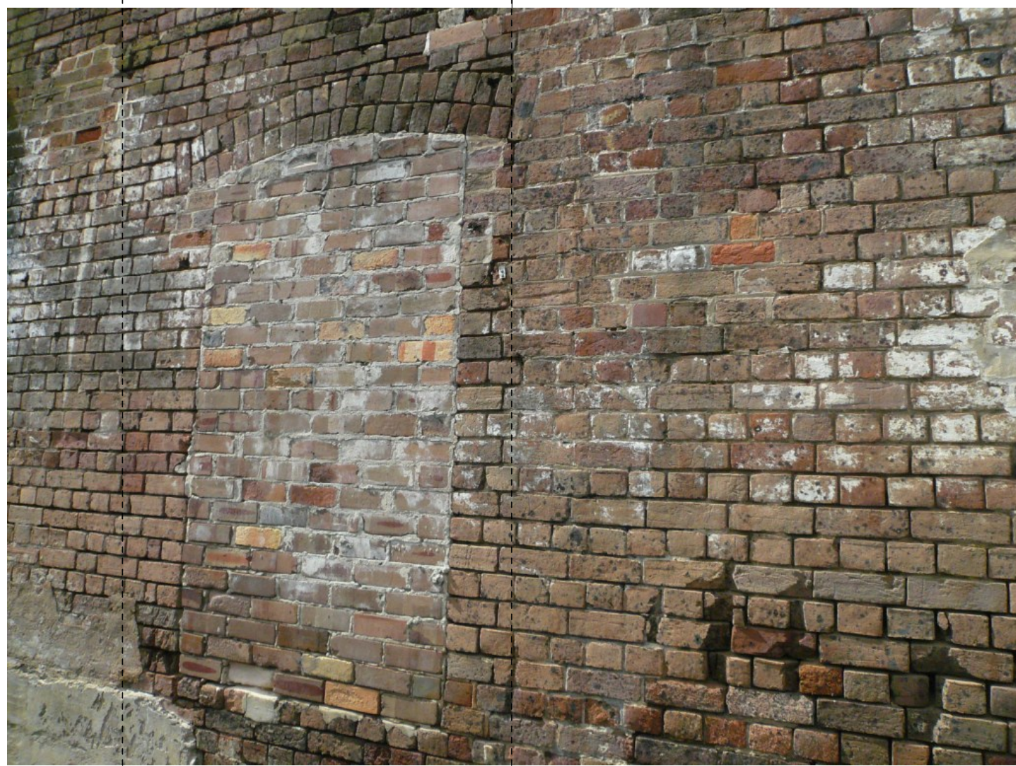
1. The proposal involves removing infill brickwork from within this arched opening in order to give residents from Block A access to bin rooms and bike storage along the southern boundary.
