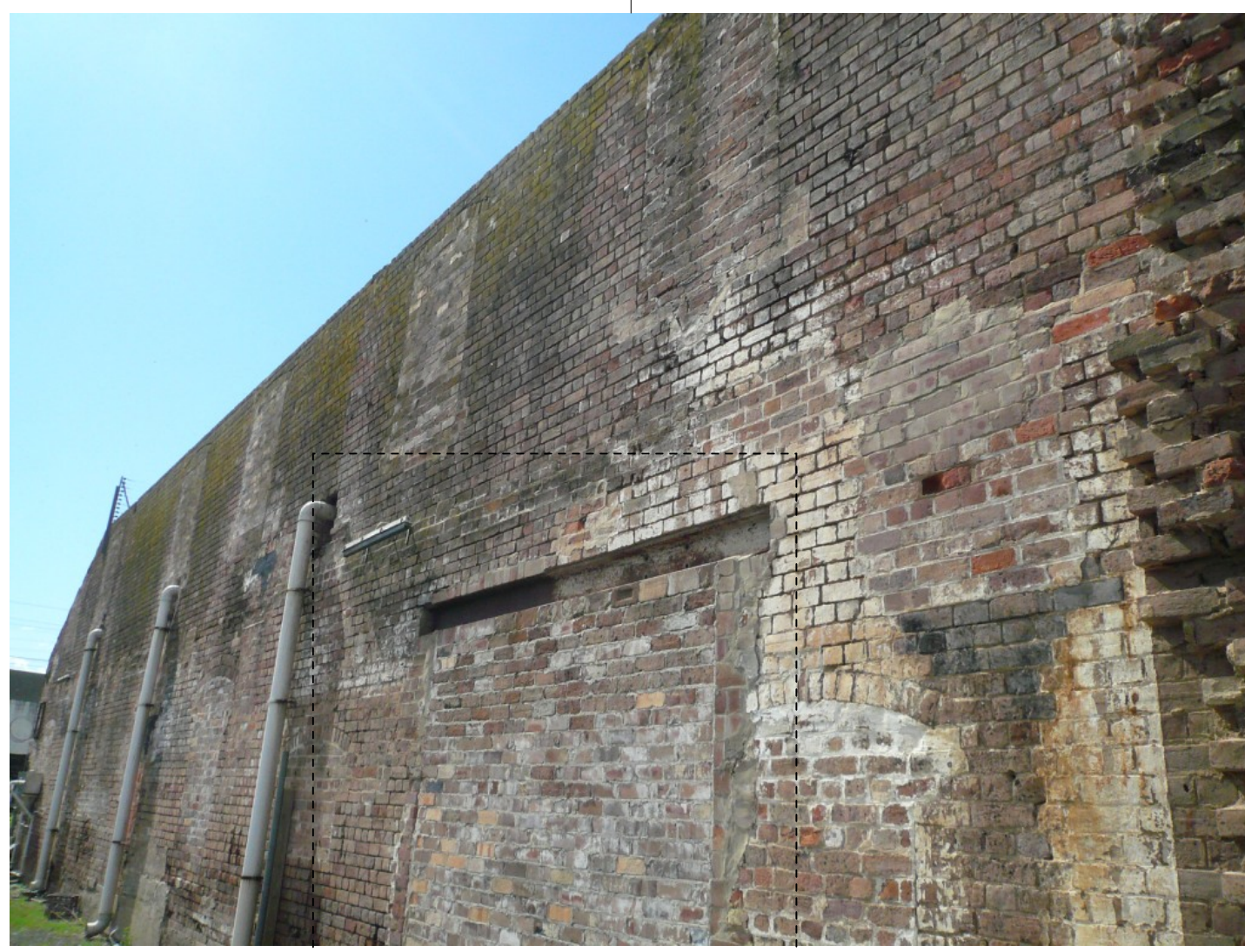
2. The proposal involves removing infill brickwork from within this square opening in order to provide a visual link from the street between Blocks A & B and the path along the southern boundary. This would improve circulation, amenity and passive surveillance on site.
